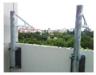
Gondola attachment structures allow for maintenance of vertical greenery that span several levels.
