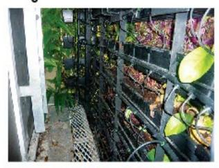
Cat ladders and sufficient space behind vertical greenery structures allow workers to effectively access the system for maintenance.
