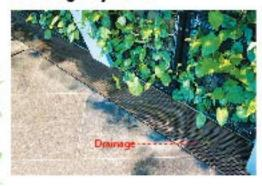
Effective drainage systems should be catered in the design of vertical greenery systems.
