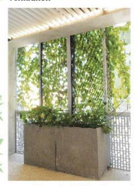
For naturally; ventilated buildings, the vertical greenery should not compromise the aggregate of the openings required.
