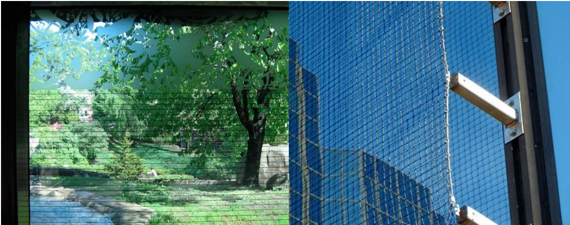
Application of a film on a glass surface facing a tract of vegetation successfully eliminated bird-window collisions (left). Netting as a bird strike mitigation strategy (right). Image credits: Philadelphia Zoo (left) and City of Toronto Bird-Friendly Development Guidelines 2007 (right)
