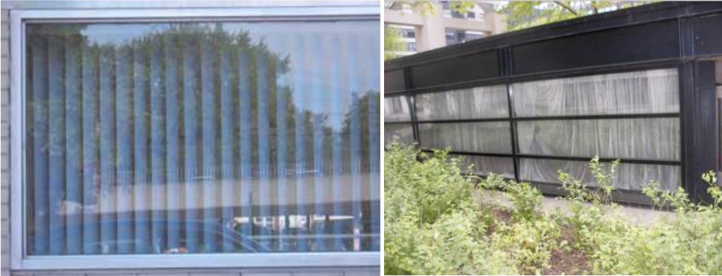
Partially open blinds (left) and curtains (right) are examples of interior elements that can reduce reflections, thereby mitigating bird strikes. Image credits: Christine Sheppard (left) and Chicago Bird Collision Monitors (right)
