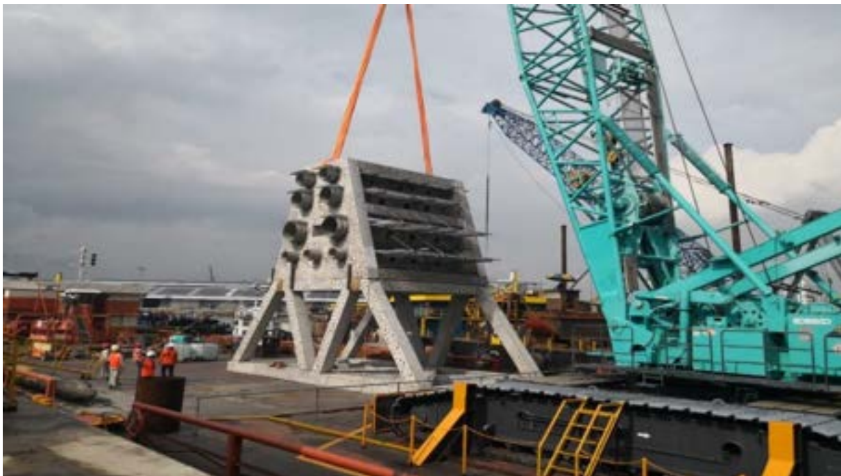
Fig. 1. Complete unit of artificial reef structure ready for installation. (Photo credit: Srirangam Santosh Kumar)
