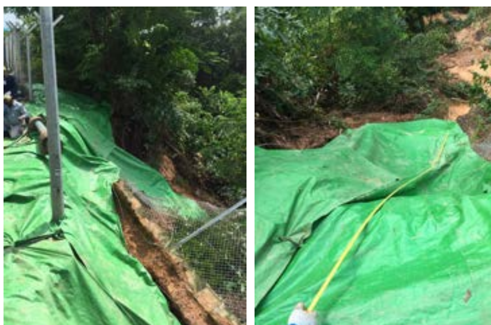
Figs. 3. Large canvas sheets were laid over to prevent the saturation of soil, which might lead to further slope failure.
