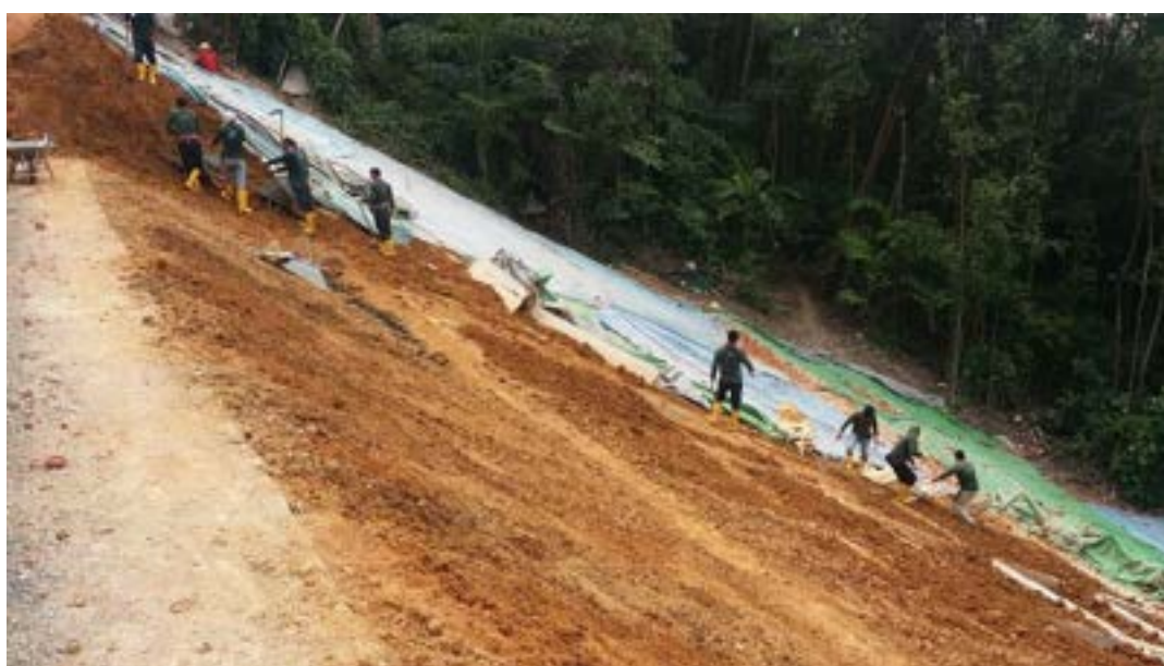
Fig. 6. Backfilling of soil in January 2017.
