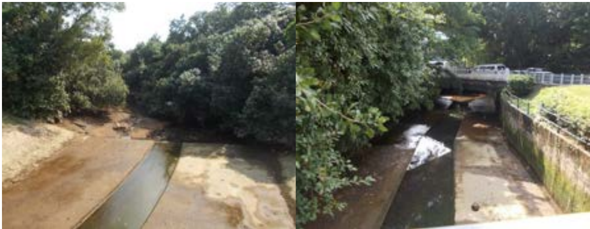
Figs. 5. Part of the Sungei Mandai mangrove that had been concretised into drains.
