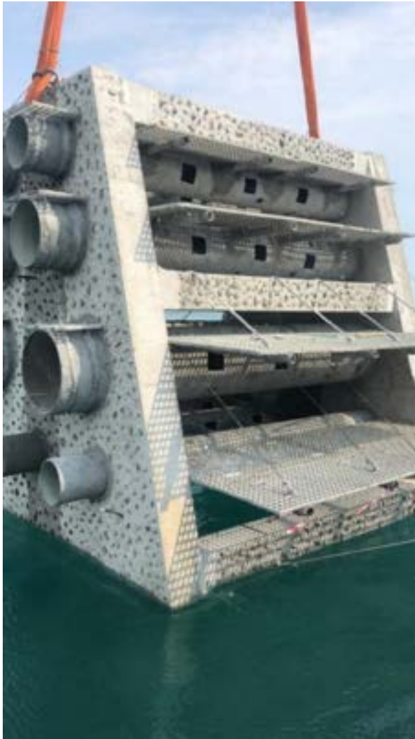
Fig. 2. Top section of artificial reef structure being lowered into the sea. (Photo credit: Srirangam Santosh Kumar)
