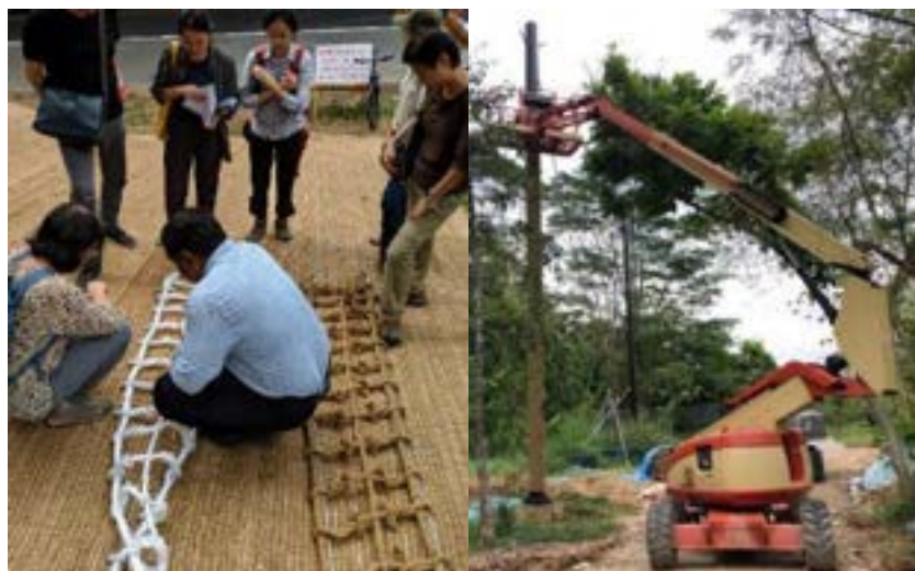
Figs. 3. Prototyping and Installation of Aerial rope bridges and Colugo Poles.
