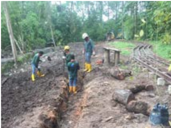
Fig. 16. Trenching of channels to bring in seawater for more areas to be inundated during high tide.
