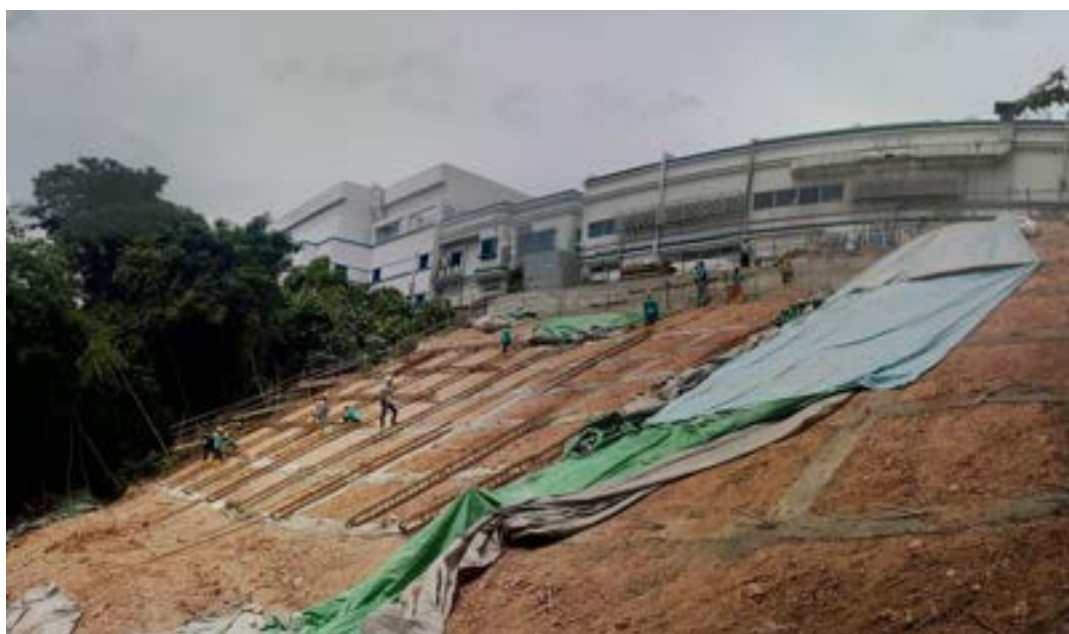
Fig. 5. Construction of grid beams in October 2016.
