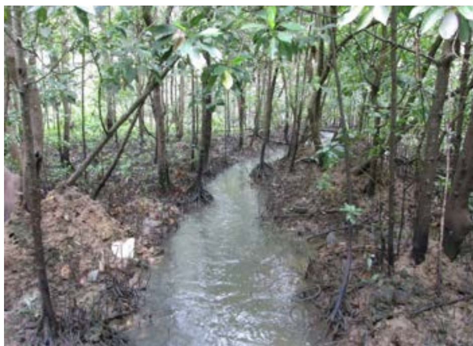
Fig. 13. Existing trench line after desilting.
