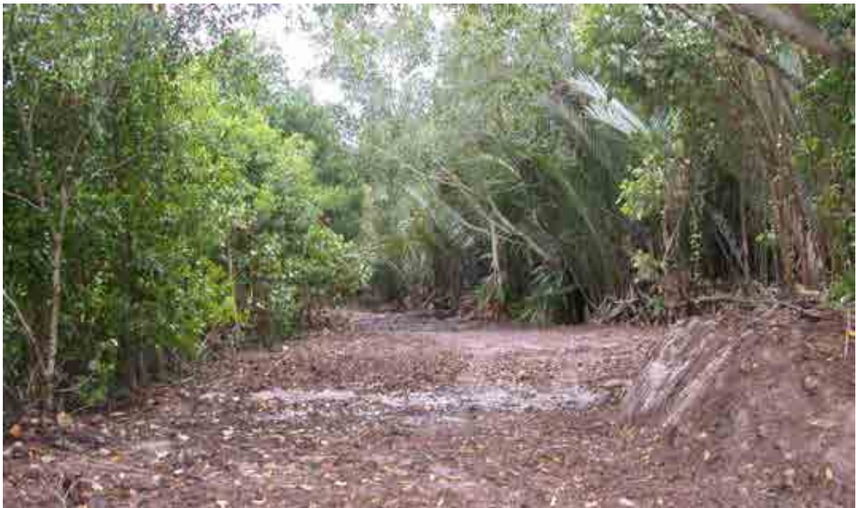
Fig. 4. Bunds around the pond were levelled down. Part of the bund yet to be cleared then can be seen on the right.
