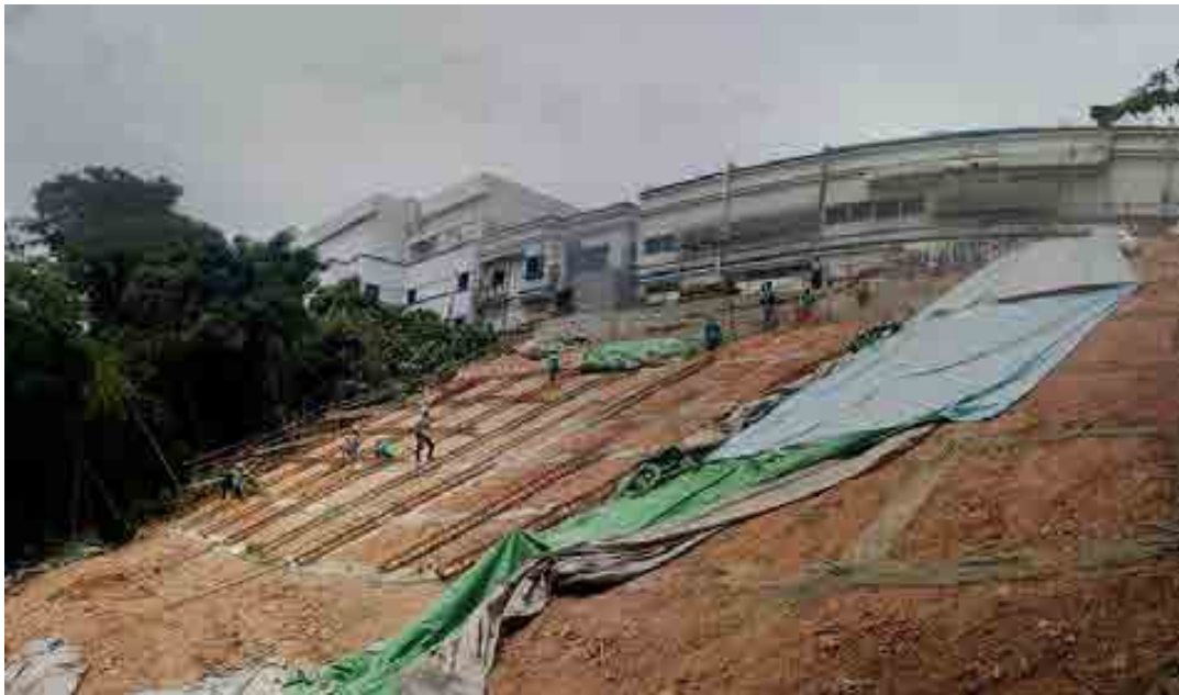
Fig. 5. Construction of grid beams in October 2016.
