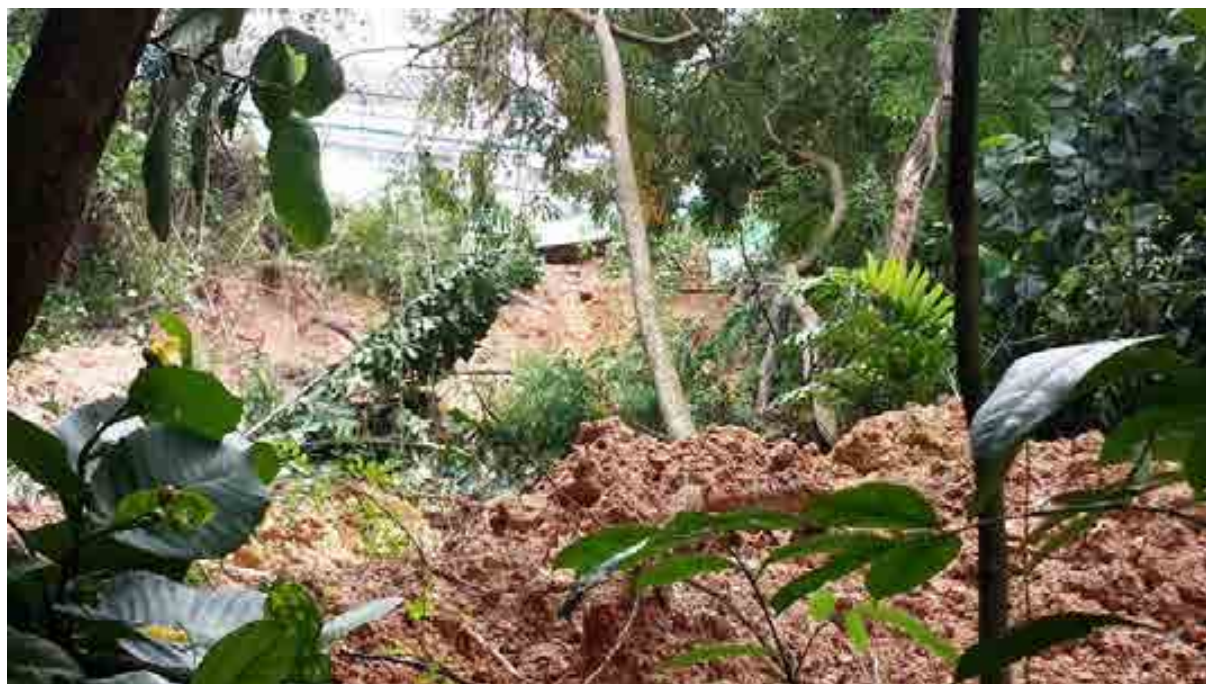
Fig. 1. Slope failure at Kent Ridge Park, Mountain Bike Trail in December 2015.
