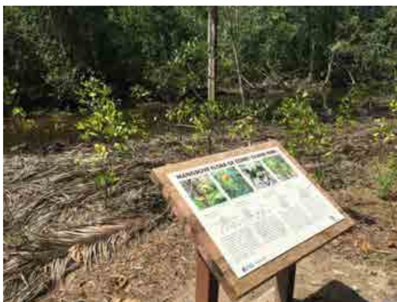
Fig. 20. Installation of educational signs.
