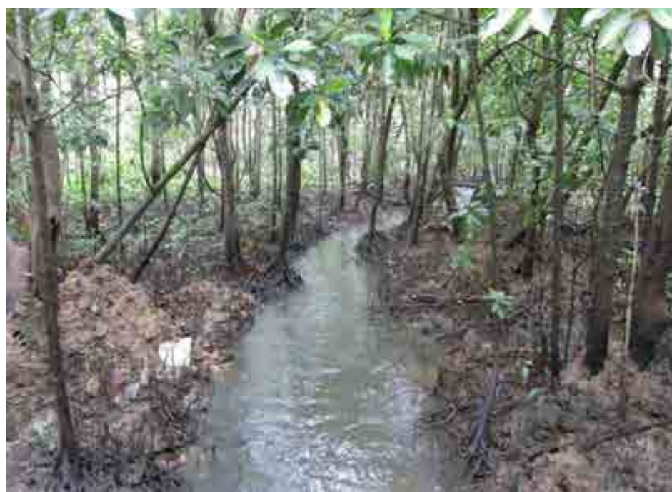
Fig. 13. Existing trench line after desilting.
