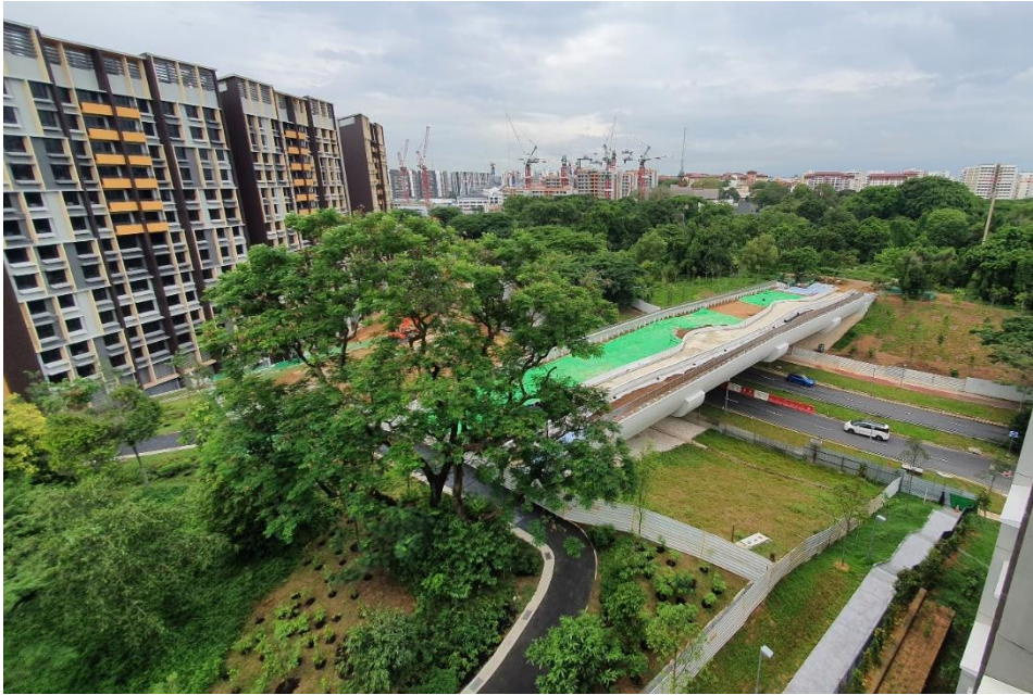
Fig. 18. View of the land bridge linking the hillock (foreground) to the main park on 21 May 2023.
