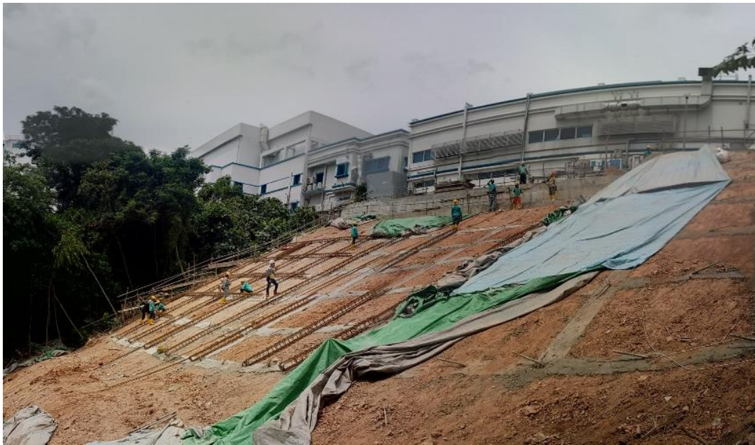
Fig. 5. Construction of grid beams in October 2016.
