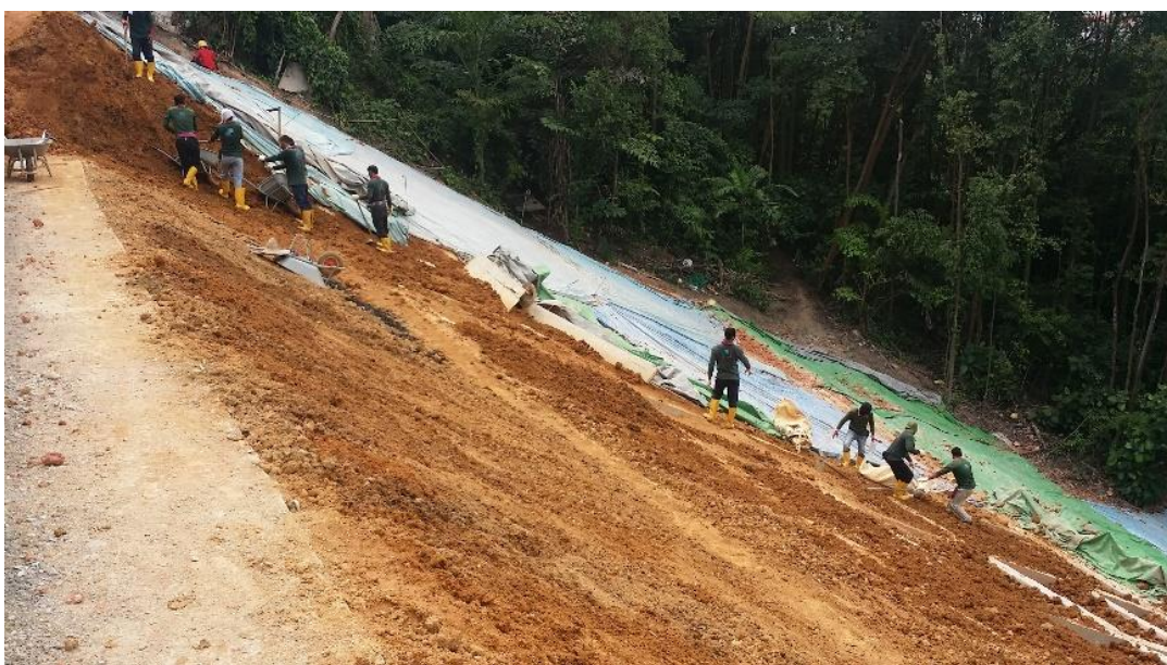
Fig. 6. Backfilling of soil in January 2017.
