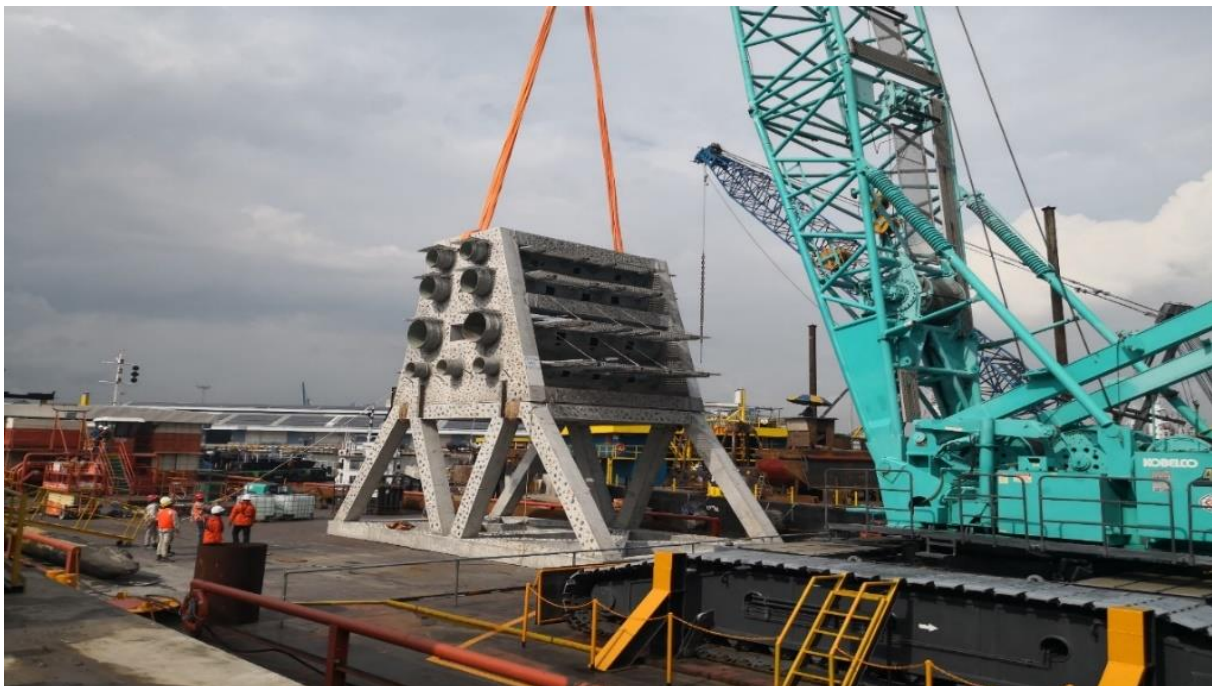
Fig. 1. Complete unit of artificial reef structure ready for installation. (Photo credit: Srirangam Santosh Kumar)
