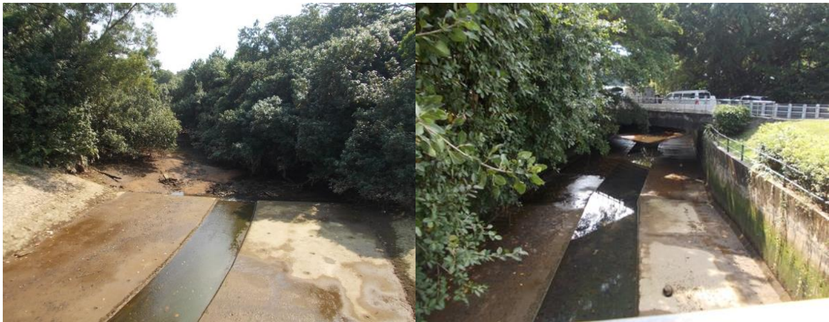
Figs. 5. Part of the Sungei Mandai mangrove that had been concretised into drains.
