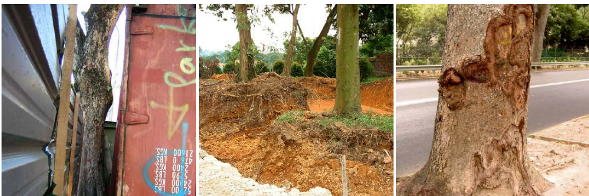
Lack of Tree Protection Zone
