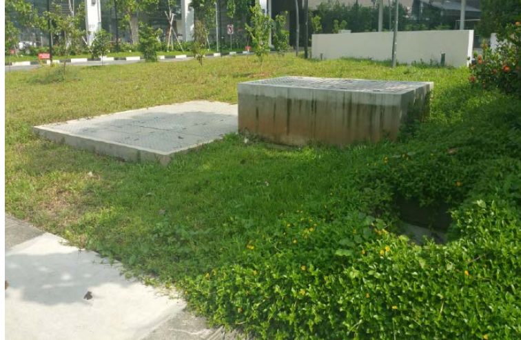
Bulk Water Meter
