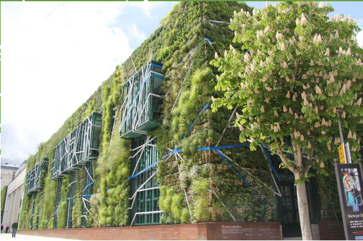
The eye-catching green facade decorates the European Congress Centre in Vitoria-Gasteiz, Spain. © Quinta fotografías
