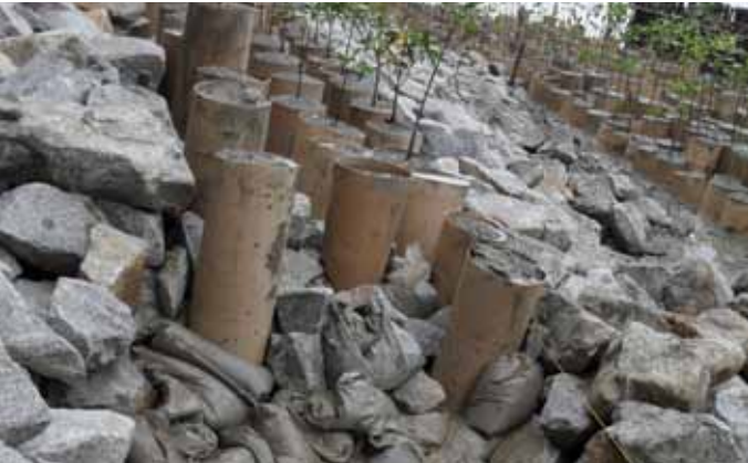
Building with nature: growing mangroves to strengthen rock walls.
