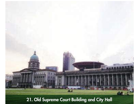
21. Old Supreme Court Building
