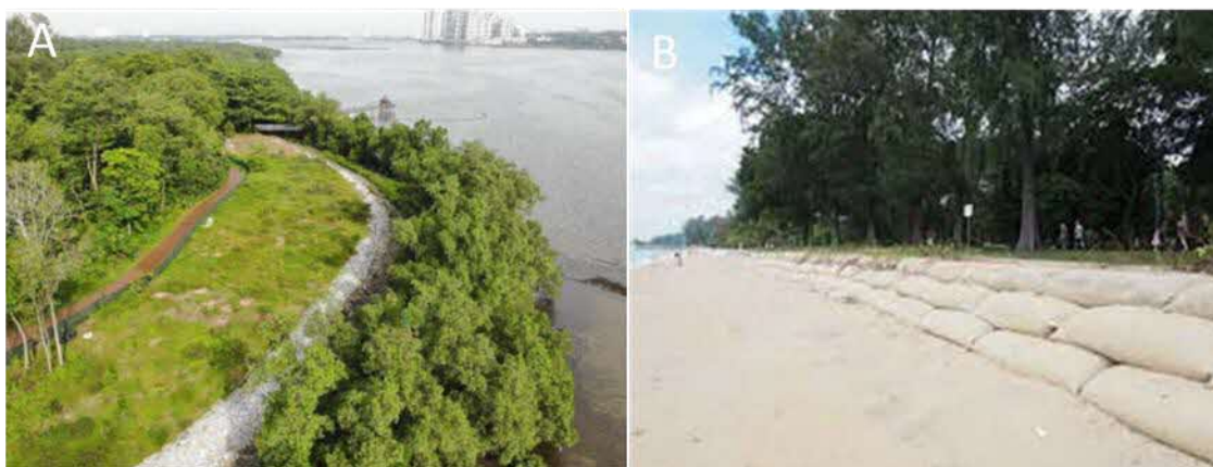
Figure 2-4. Photographs of the existing coastal protection works used in Singapore: a) Kranji Coastal Nature Park 2 , and b) Geobags applied at East Coast Park (NParks) 3
