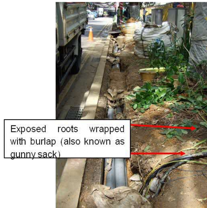
Figure 9: Tunneling under roots.
