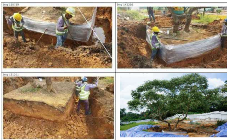
Transplants: Determining root ball size, shaping root balls, protection with polythene wrap to prevent excessive desiccation and anchoring trees prior to transplant.
