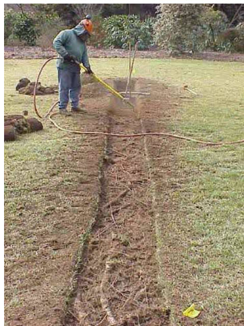
Figure 10: Root exploratory works using an air spade. Air spading avoids damage of structural and even feeder roots of the tree.
