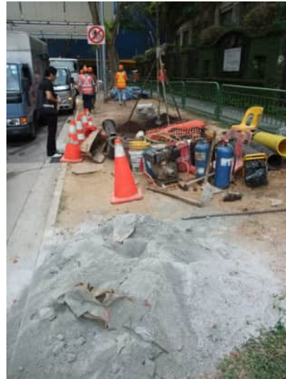
Figure 2: Construction material and heavy machinery are prohibited within the TPZ
