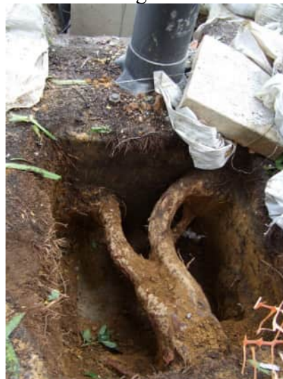
Figure 3: Trial trench by skilled workers using hand tools exposing root architecture
