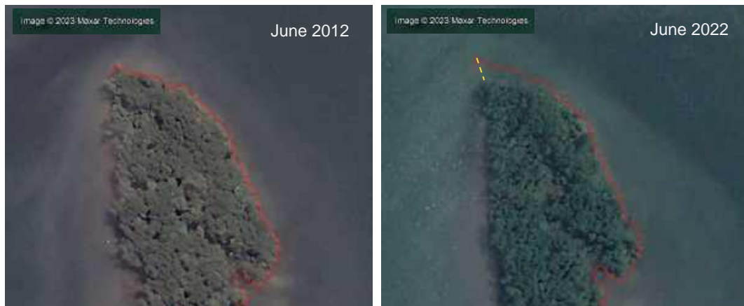
Figure 5.9. Area of focus B. Northwest point of Pulau Ketam with signs of erosion from June 2012 to June 2022. The largest deviation from the 2012 shoreline is approximately 24 m, indicated by the yellow dashed line
