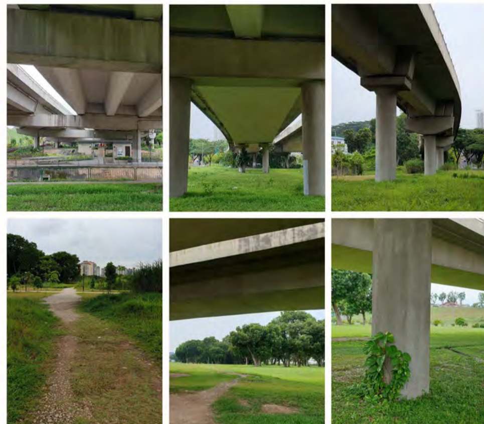
Existing site conditions
