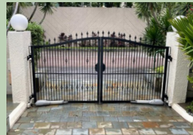
Modify the gates/fences to make the gaps in fences smaller
