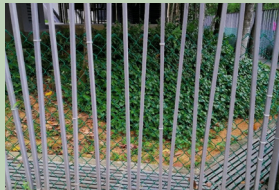
Wire mesh to cover gaps in gate
