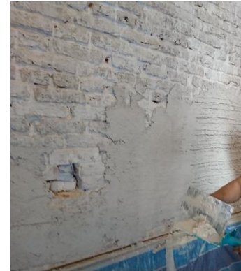
Brick wall with cement plaster finish
