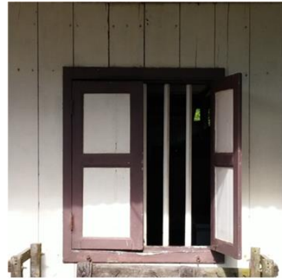
Timber frame and timber louvered/panel windows/ timber stile and rail
