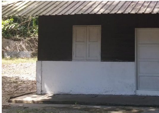
Cement Plaster wall
