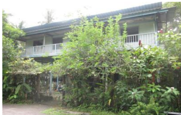
Double-storey kampung house
