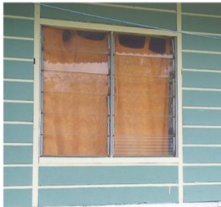
Mild steel framed glass casement windows or with glass/metal louvres
