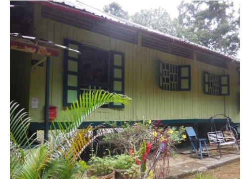
Partially elevated house
