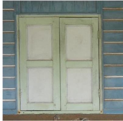
Timber frame and timber louvered/panel windows/ timber stile and rail
