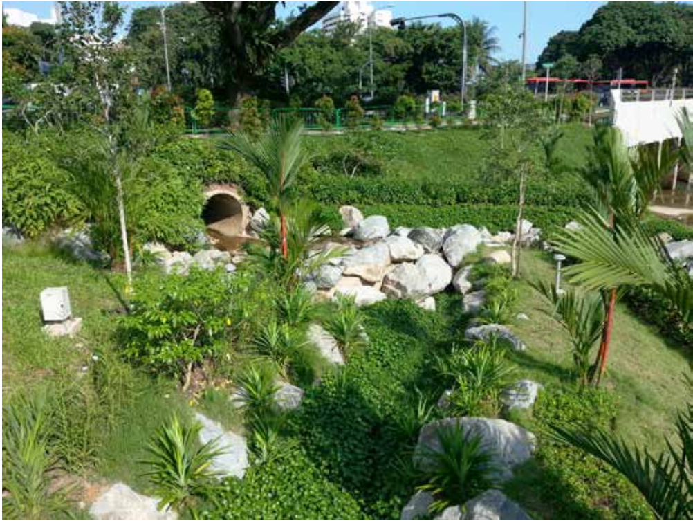
Figure 25. Hybrid vegetation planting along a canal in Ulu Pandan that incorporates natural stream elements. (Photo: A.T.K. Yee).
