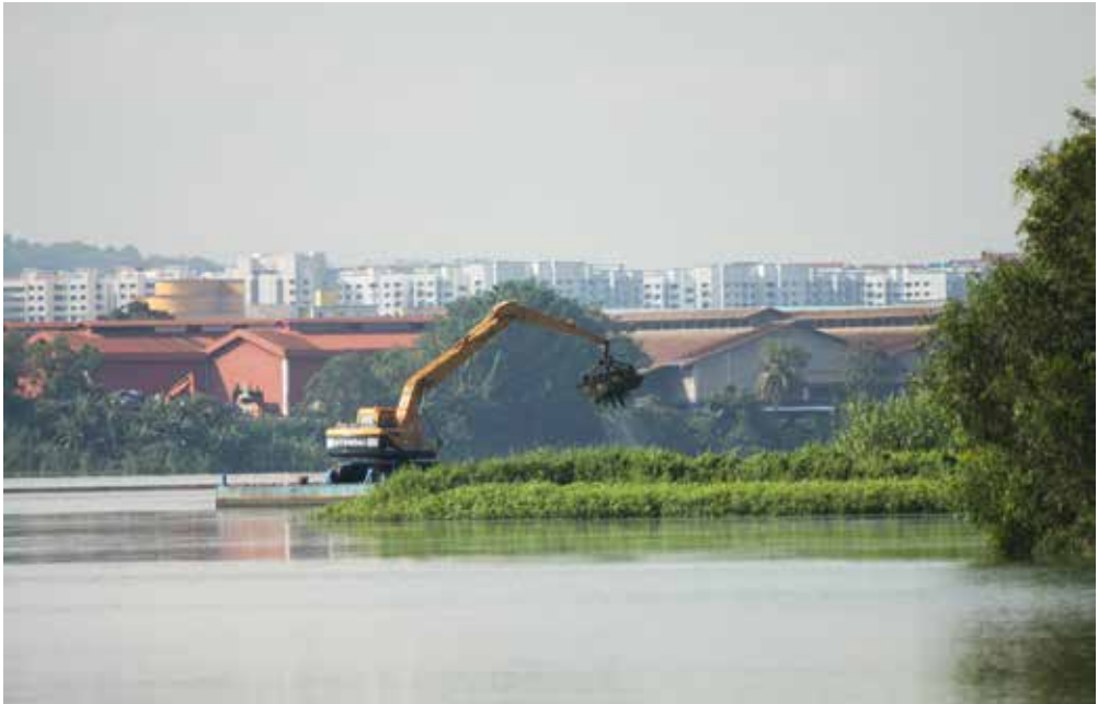
Figure 15. Open waters at Kranji Reservoir, where aquatic plants are regularly dredged. (Photo: K.Y. Chong)
