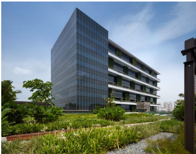
Photo credit: SAA Architects Pte Ltd
