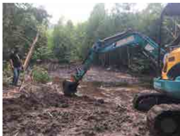
Fig. 15. Regrading of soil to lower the ground level for more areas to be inundated.
