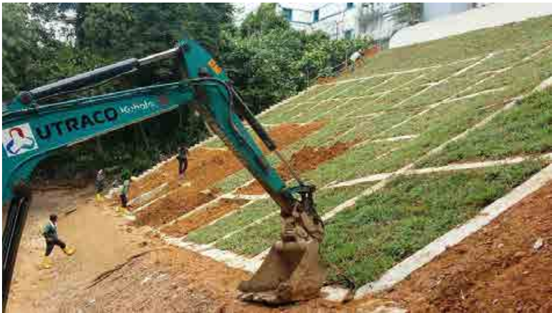
Fig. 7. Planting of turf at end January 2017.
