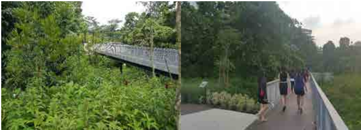
Fig. 4. A boardwalk cutting through the secondary forest has also been installed at Fusionopolis South to allow visitors to get closer to nature.
