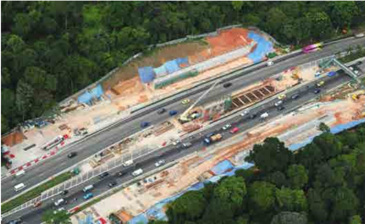
Fig. 2. The traffic flow along the BKE was maintained throughout the construction phase, while the inconvenience for the commuters along BKE was minimised.
