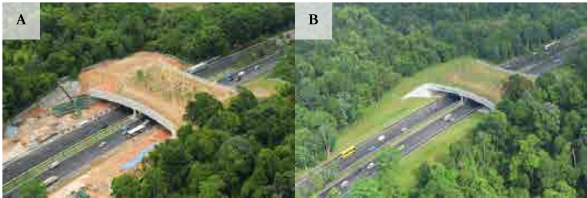
Figs. 6. Aerial photographs of the Eco-Link@BKE project taken in (A) November 2013 and (B) June 2014.
