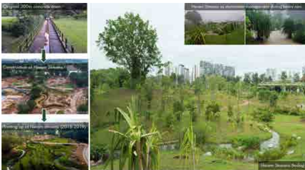
Fig. 11. Creation of Neram Streams by transforming a 300-metre concrete canal into a series of braided, naturalised and vegetated streams.
