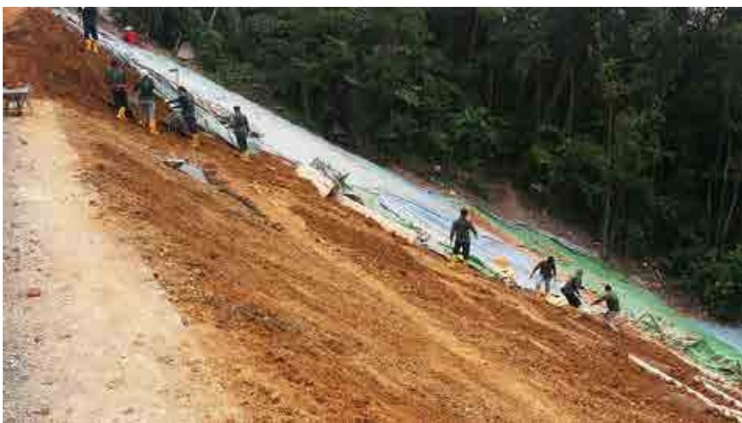
Fig. 6. Backfilling of soil in January 2017.
