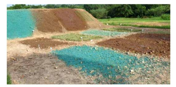
**Fig. 3** Experimental plots after one week of hydrosprigging application using both coco peat slurry (brown) and Terramatrix mulch slurry (green)
