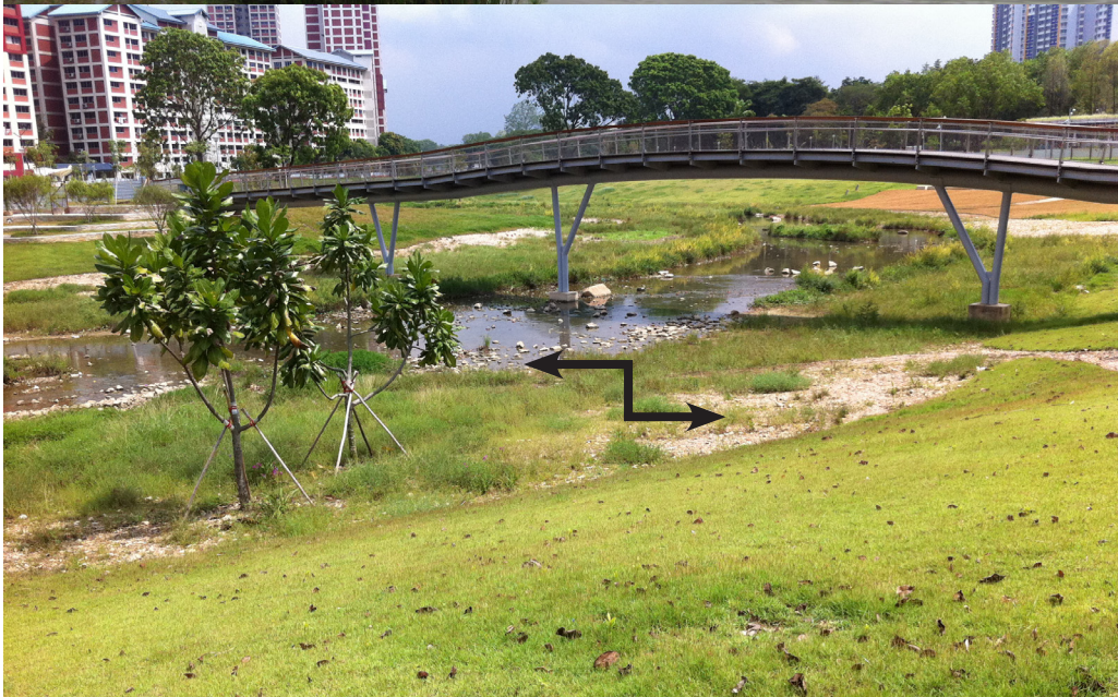
Fig 5. The naturalised canal in Bishan Park (wet soil condition indicated by arrow)
