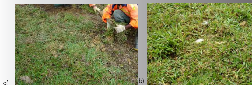
Figure 2. a) Planting by close turfing. b) Post plant topdressings and rollings are required to prevent an uneven turf surface.
