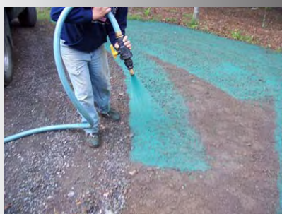
Figure 5. Planting by hydroseeding
