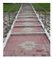
In this flight of steps, the designer simply spread out the threads evenly throughout the entire grade change, resulting in a series of non-ergonomic steps. They do not conform in dimension to the average human stride.
