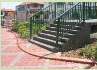
An irregular riser within a very long and consistent flight of steps can be especially disconcerting as it is totally unexpected.
