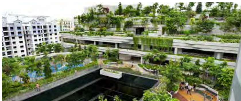
Stacked "club sandwich" approach effectively houses multiple facilities in a small site footprint of 0.9 hectares whilst ensuring green vistas from various vantage points. Image by Patrick Bingham-Hall
