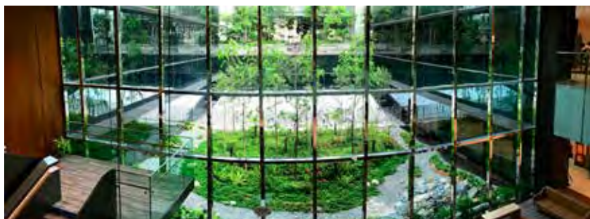
Landscaped terraces create a continuous curtain of greenery that cascades from the top to the bottom of the development. Images by Ramboll Studio Dreiseitl Singapore Pte Ltd
