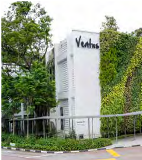
Free-flowering climbers grown around the building premises help to soften its outlook and create pocket habitats for wildlife. Image by National University of Singapore
