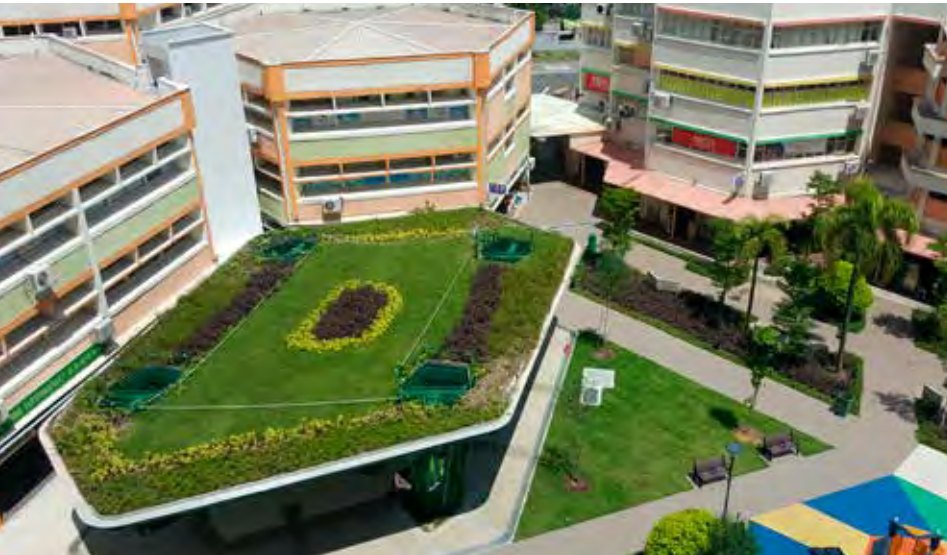
Green roofs are a simple but effective way to dress up concrete structures and reduce cooling costs. Image by Interconsultants Pte Ltd
