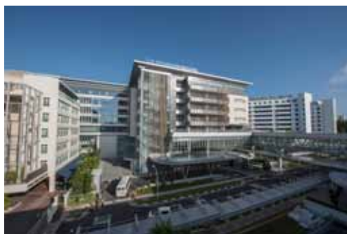
The Integrated Building was designed to optimise patients' recovery and independence (Photo: Changi General Hospital and Eastern Health Alliance).
