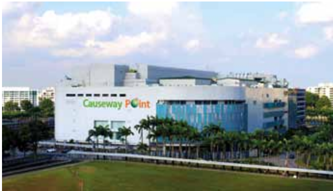
Causeway Point has easy-to-read signages and family-friendly amenities (Photo: Causeway Point).
