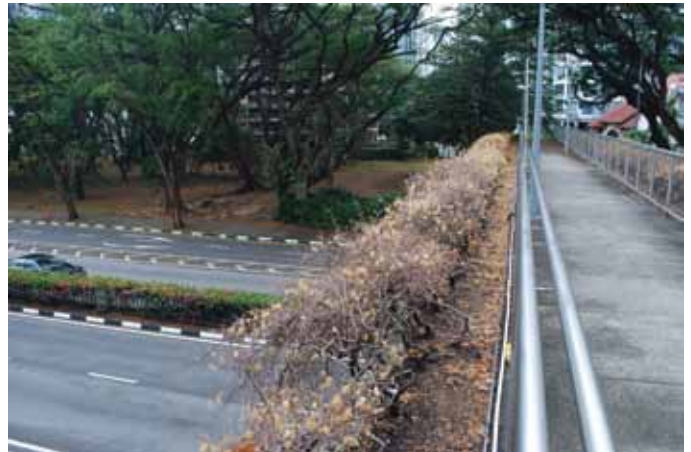
10. Dry amenity planting at a pedestrian overpass at Newton Circus.
