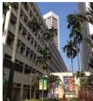
Connection One, government office building, Green Mark Platinum award.
