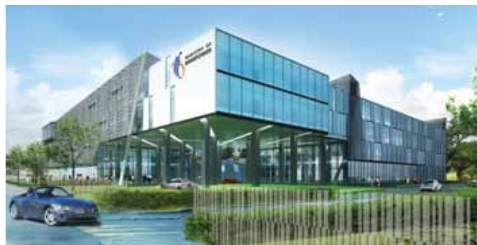
Ministry of Manpower Bendemeer Services Centre, government office building, Green Mark Platinum award.
