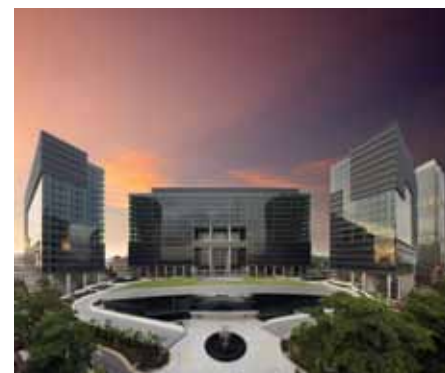
Mapletree Business City, private office building, Green Mark Platinum award.
