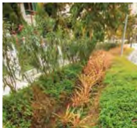
2. Vegetative swales in The Rainforest condominium filter pollutants from groundwater (Photo: City Developments Ltd).
