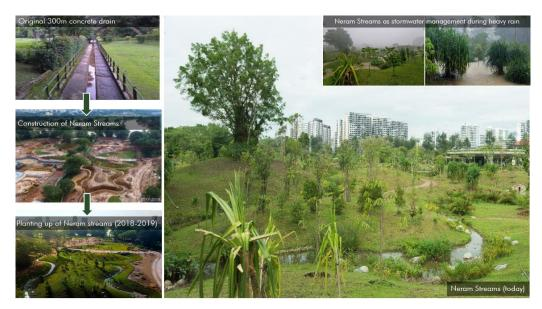
Fig. 11. Creation of Neram Streams by transforming a 300-metre concrete canal into a series of braided, naturalised and vegetated streams.
