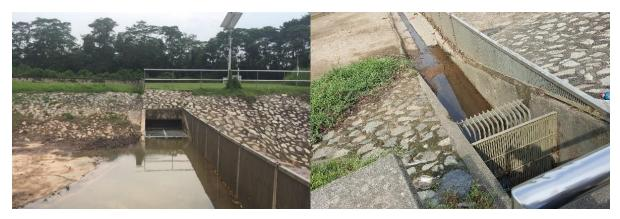
Figs. 8. A filtration system at the start of drain channels into the mangrove area.
