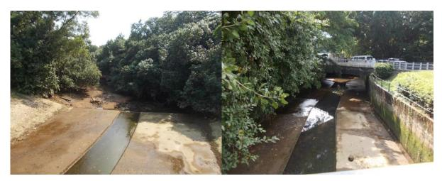
Figs. 5. Part of the Sungei Mandai mangrove that had been concretised into drains.
